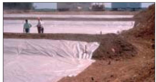
2. Earthen berms (if used) between infiltration beds should be left in place during excavation. These berms do not require compaction if proven stable during construction (Cabill Associates Photo)
