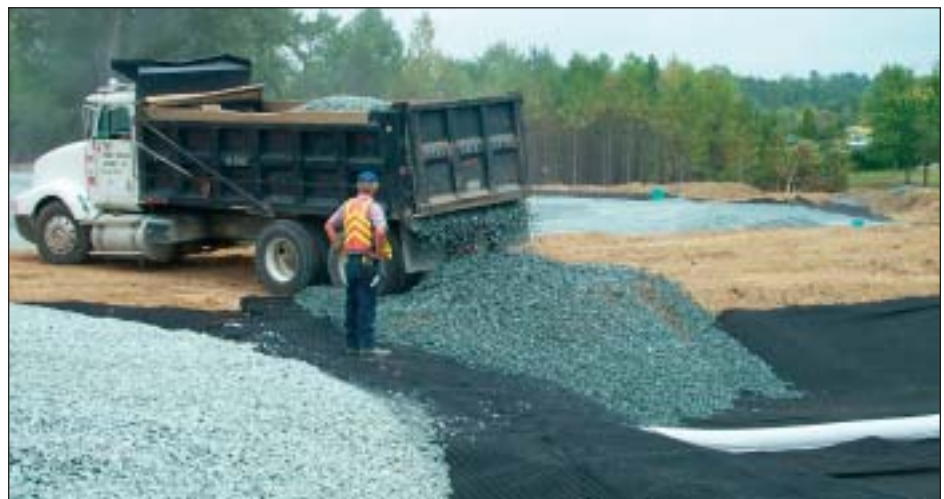
2. Earthen berms (if used) between infiltration beds should be left in place during excavation. These berms do not require compaction if proven stable during construction (Cabill Associates Photo)
