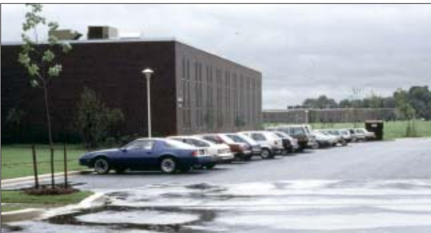
6. The finished surface looks like conventional asphalt—until it rains. Infiltration beds are completely under the parking lots, minimizing the disturbance envelope. (Cabill Associates Photo)
